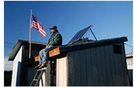
Pamela Kliment Solar Panels at Nickelsville 637pm
